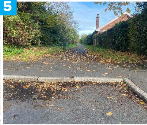
5 A resident has asked if dropped kerbs can be installed between Birch Avenue and Oak Avenue to help people with wheelchairs, buggies or mobility issues.
