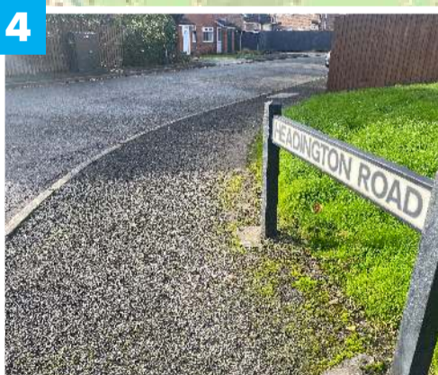
4 We've asked for the 'gully sucker' - yes, that's its name, to attend to block grids, including Headington Road, following requests from residents.
