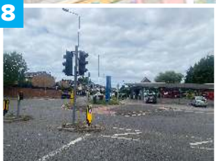
8 It might be one of the longest residential roads in the Borough, but Millhouse Lane has no road sign at the junction with Hoylake Road. We've asked for one!
