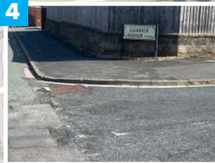
4 Residents asked for the junction markings at Garrick Avenue to be repainted. We've reported this to the Highways Department and await their response!
